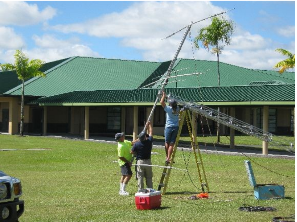
Antenna engineers at work
